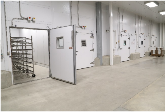
Figure 6: Blast Freezers
