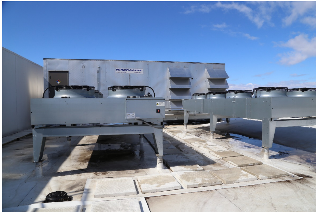
Figure 5: Rooftop-Mount Rack House
