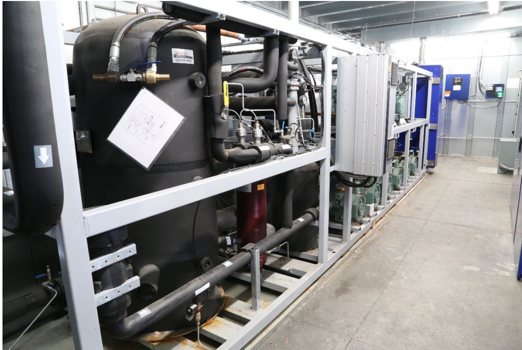
Figure 4: Hillphoenix Advansor CO 2 Transcritical Booster System
