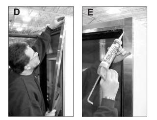
**E.** Reinstall the J-strip with the screws and apply a new bead of clear silicone to seal the J-strip to the edge trim.
