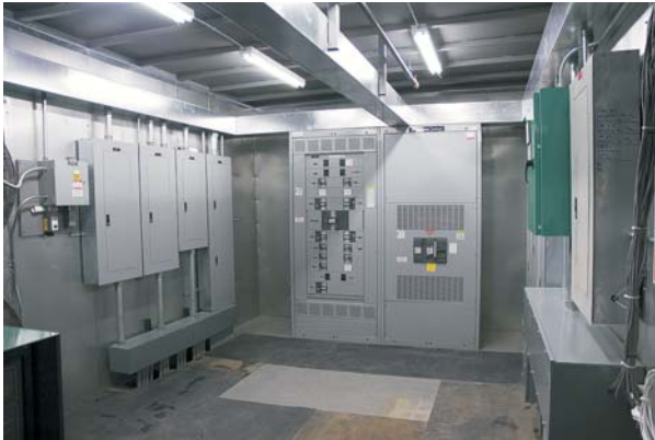
A Combination Center in the above and below photos show electrical and mechanical distribution sections.
